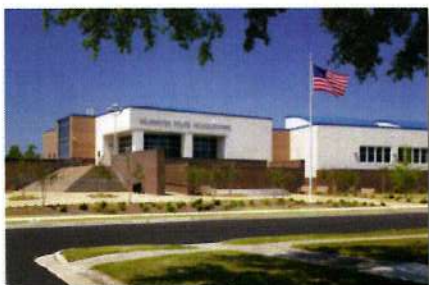
Wilmington Police Headquarters Wilmington, NC
